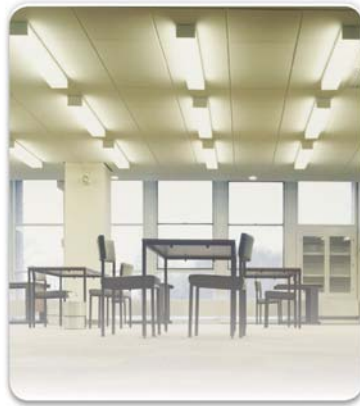
Linear Fluorescent Ballasts
