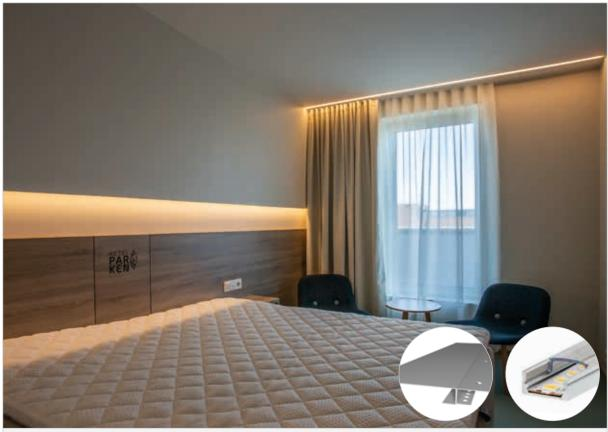
Profile over the bed: SNL // Profile in celing: A1 Standard // LED-strips:  $9{,}6W/m$
