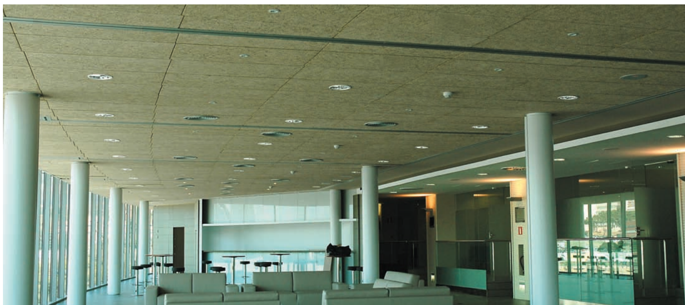
VIP & LOUNGES AREA F.C. BARCELONA STADIUM. Barcelona
