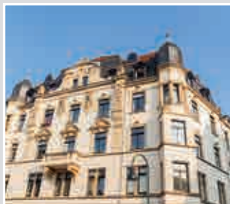
Historically significant facades in exposed masonry or stucco facades
