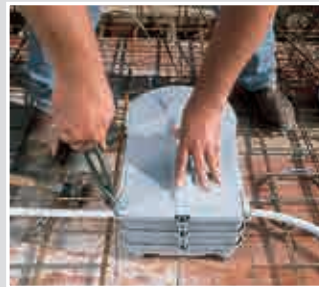
Also secure the housing to the reinforcement.
