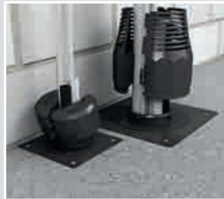
Place sealing cylinder around the cables or conduits and then snap into place with the sealing cylinder.
