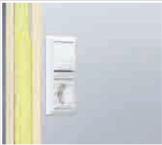
Example of installation of a switch/socket combination.
