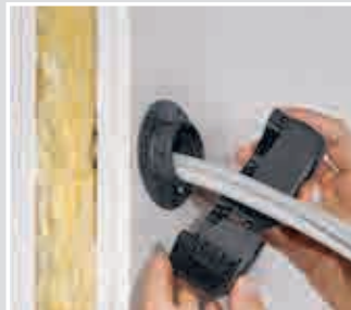
Open the sealing element and remove it.
