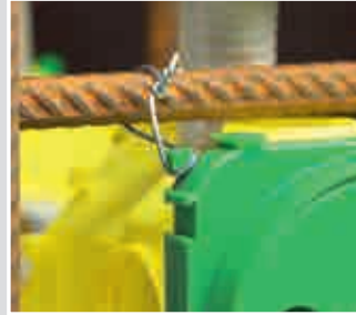
Tie lugs provide additional security if extreme loads are expected.
