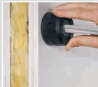
Place the sealing element on the seal cylinder and secure it with a 1/4-turn (bayonet fitting).
