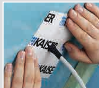
Stick on the sleeve and press firmly on to the base, working outwards from the centre.
