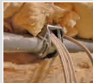
The mast which supports the parabolic mirror must also be incorporated in the equipotential bonding.
