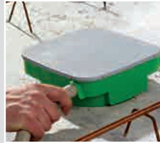
Insert conduits and concrete up.
