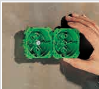
Attach front part to formwork.
