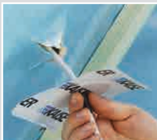
Push the sleeve over the cable or conduit.
