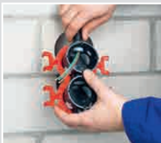
Creating installation opening.
