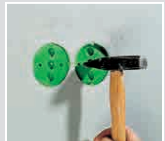
Open concrete building boxes or casings, then fit equipment or cover.
