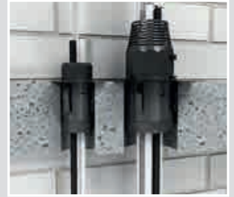
Two ceiling penetration sealing systems for different applications.
