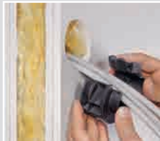
Place the two-part sealing cylinder around the cables and press together.
