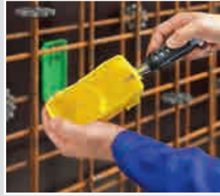
Use the KAISER punch pliers or the opening cutter to make exact cable or conduit entries.
