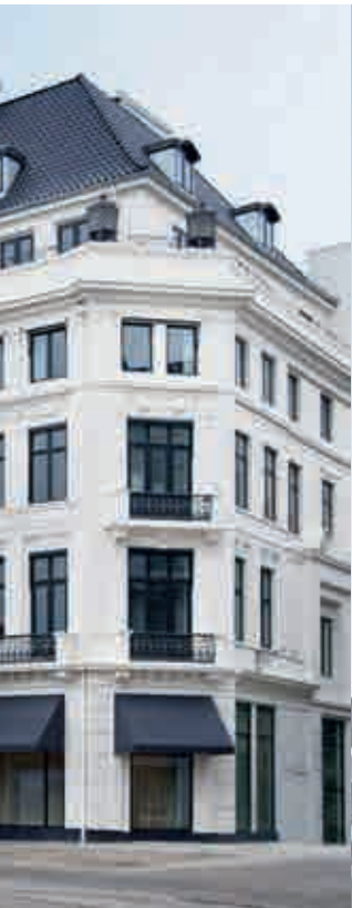
SALEWA headquarters | Bolzano, Italy
