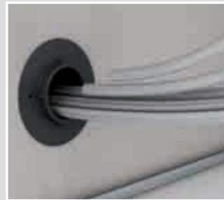
Insert the new cables and conduits.
