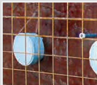
Fasten to the formwork using tensioning wire and nails.
