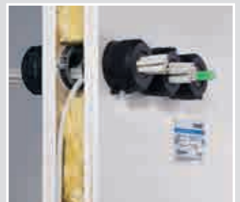
This ensures sealing and the necessary room separation.
