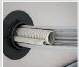
Feed sheathed cables and conduits through the sealing cylinder.
