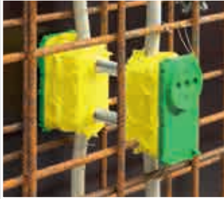
Opposing installation, cable entry behind the reinforcement.
