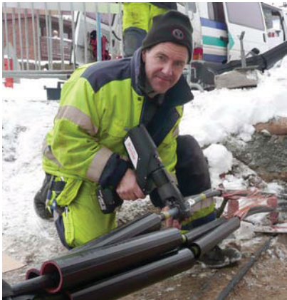
Crimping with Elpress crimp tool PVL1300.
