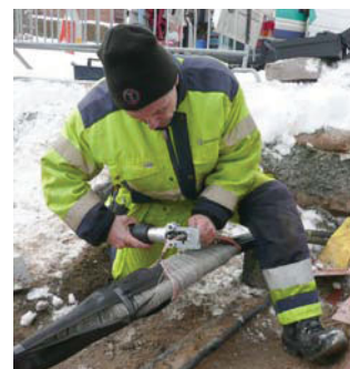
Crimping with Elpress crimp tool PVL611.
