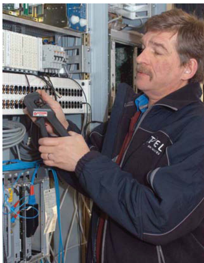
Elpress Mobile, a professional crimp tool with interchangeable dies.
