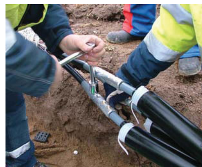
Bolts are tightened using a wrench. It is also possible to use a battery operated wrench.
