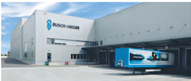
Logistics Centre at the headquarters in Lüdenscheid
