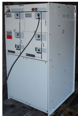
From IAC-test with arc suppressor 20kA/1s
